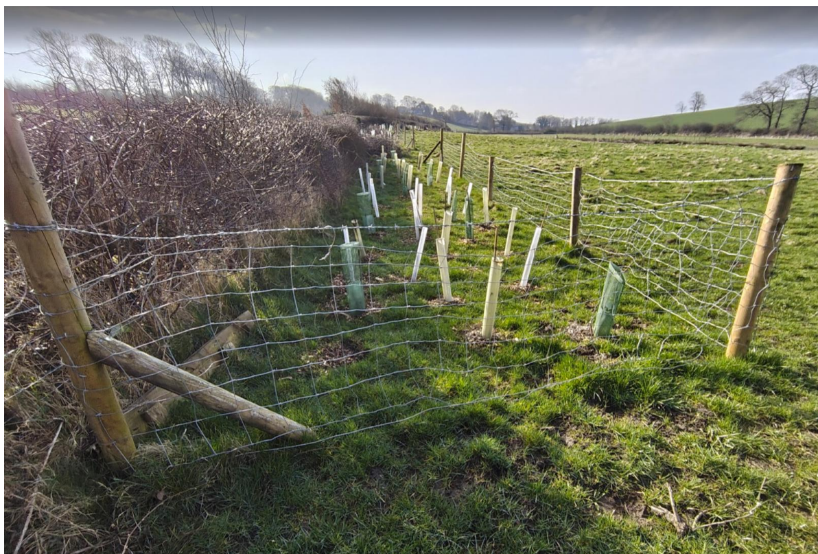
Figure 3 – Example of a strut, and insufficient tensioning in a fence without strainer posts
