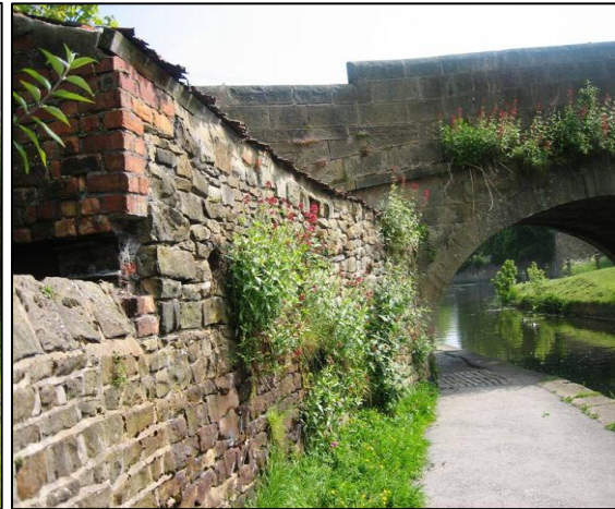
Side elevation built into the boundary wall
