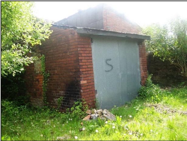
Second Building: Modern Brick Work to the front, older brick work to the rear
